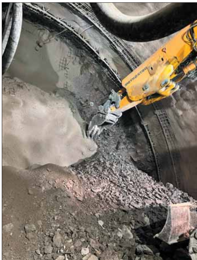
Obr. 5 Razenie kaloty v TT5a Fig. 5 Top heading excavation in TT5a
